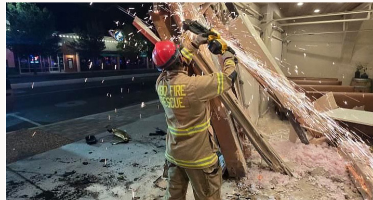
Crews clean up a scene after a vehicle struck a building at 3423 Central Ave NE on 10/2.
